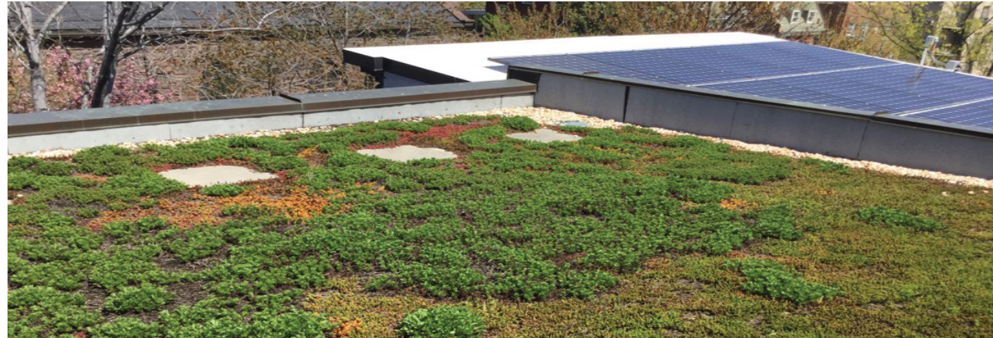
FCNL's buildings features 27 solar panels and a living roof, covered by sedum plants. Photo by Furbish Co.
